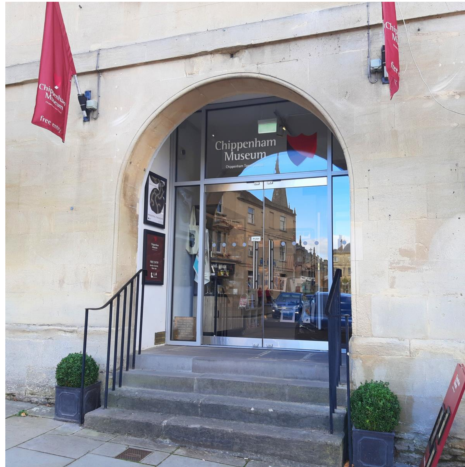
This is the main entrance to the museum. It has four steps up to glass doors, which you push open.
